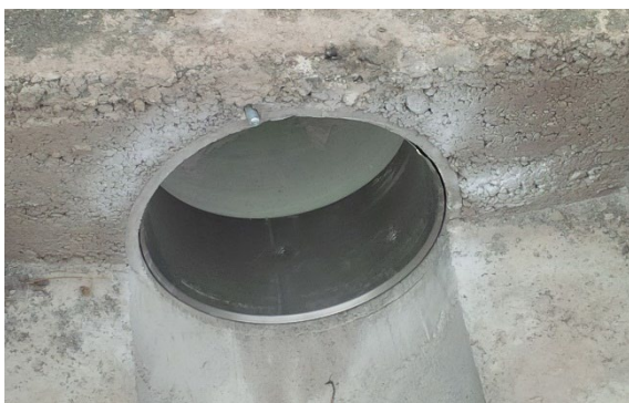
Figure 20: Liner connections with Pipe-Seal-End
