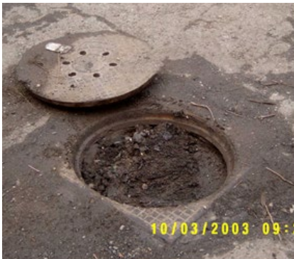
Figure 28: Shaft fouling
