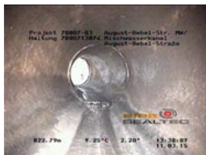
Figure 14: Axial change of direction
