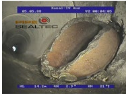
Figure 15: Protruding connection piece
