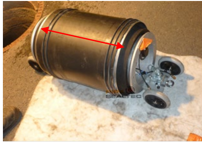
Figure 53: Positioning the prepared stainless steel sleeve on the packer
