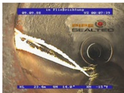
Figure 18: Penetrating roots
