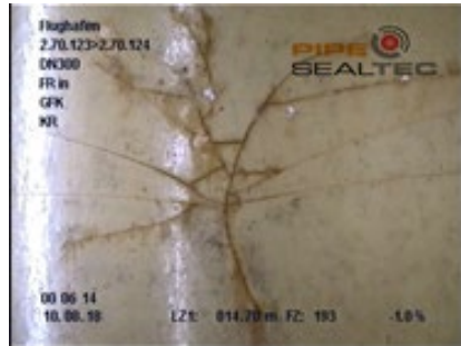
Figure 12: Crack formation
