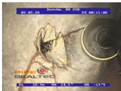
Figure 11: Pipe outbreak
