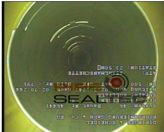
Figure 82: Documented rehabilitation area Pipe-Seal sleeves Serial mounting
