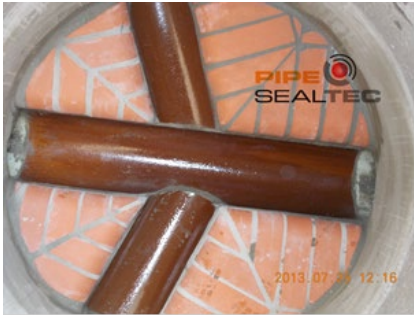
Figure 26: Forming of access possibilities such as channel profile and pipe connection
