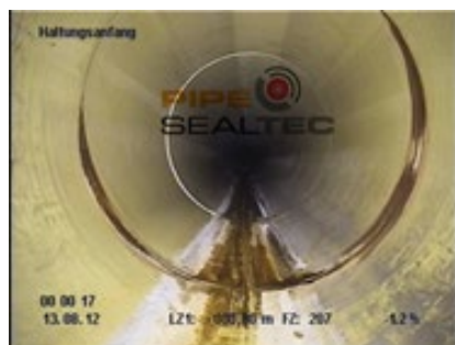
Figure 13: Leaky pipe connection
