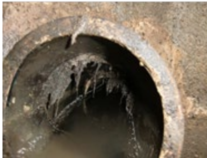
Figure 19: Penetrating roots
