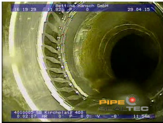
Figure 87: Rehabilitation with Pipe-Seal-Flex on angular offset
