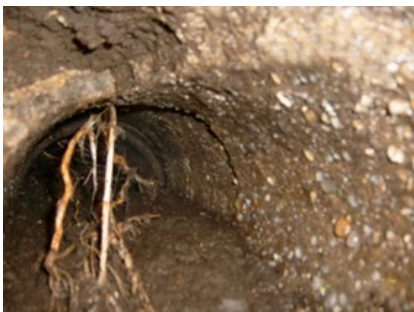
Figure 29: Pipe fouling
