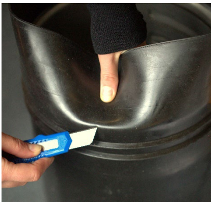
Figure 49: Simple cut of overlapping rubber
