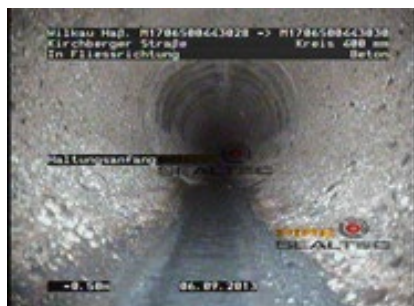
Figure 17: Concrete corrosion
